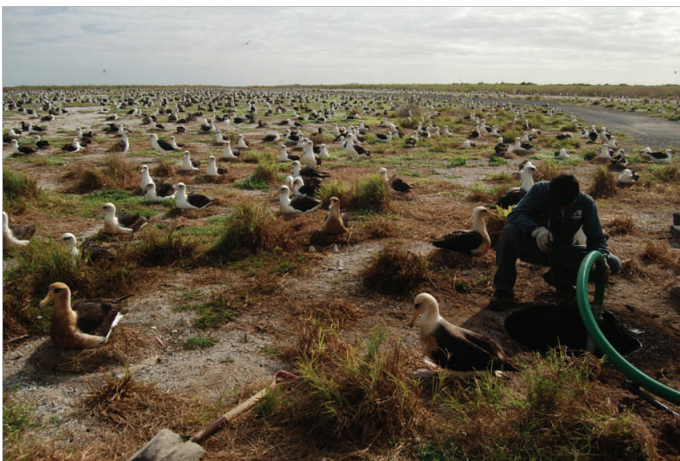
Chugach Industries staff working to pump oily water out of abandoned line. Note impacted albatross in left foreground.
