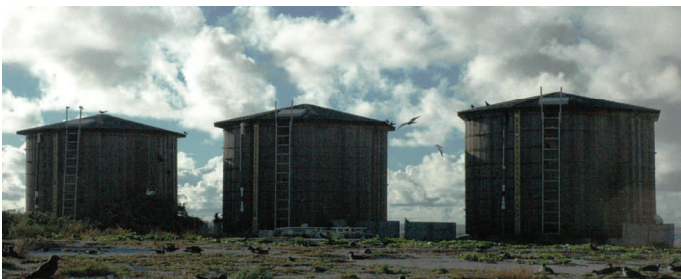
Three water tanks/cisterns on Tern Island hold the "community's" freshwater supply.
