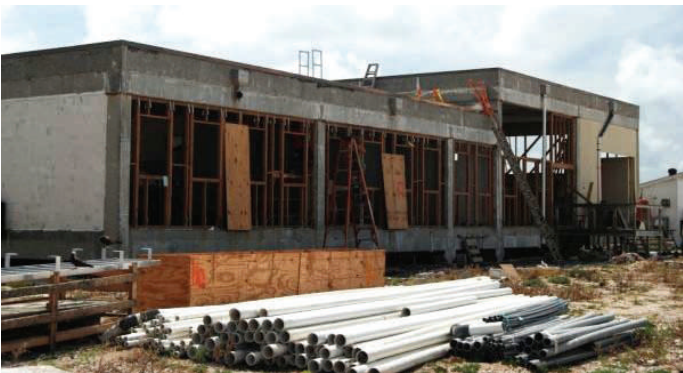
Replacing "blow-out walls" with permanent walls in Tern Island's storage warehouse.
